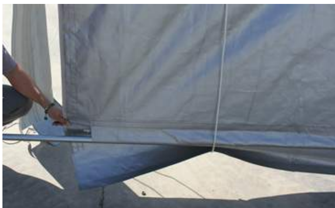
Step 1: Insert the door dropping tube (part #21) into Pocket along Bottom edge of Roll Up Door.
